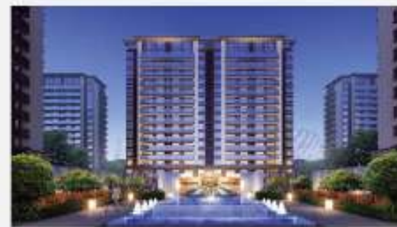
FUJIAN Fujian Sunshine Industrial Development
